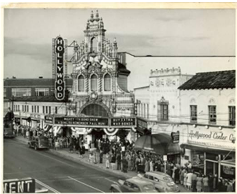
The Hollywood Theatre with the Arcade building to the west.
